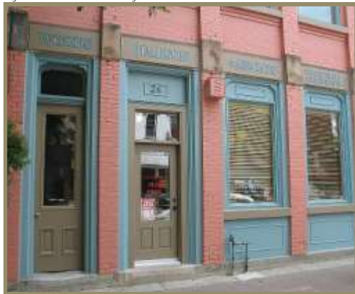
Woods Pearson & Associates, 26 Front Street West in Strathroy after extensive renovations and assistance from a Main Street Middlesex Façade Grant.
